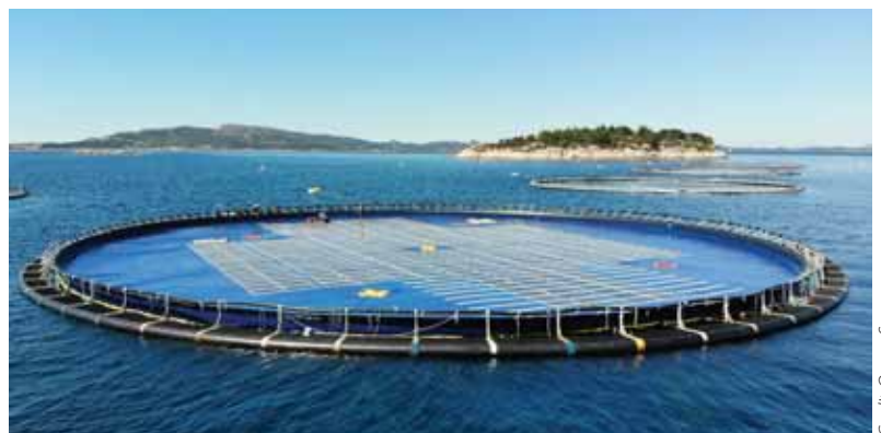
A previous floating solar test system installed by Ocean Sun off the coast of Norway .
