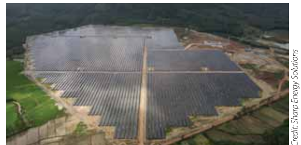
Sharp Energy Solutions's latest 50MW installation will take it total installed capacity to 340MW in Vietnam.
