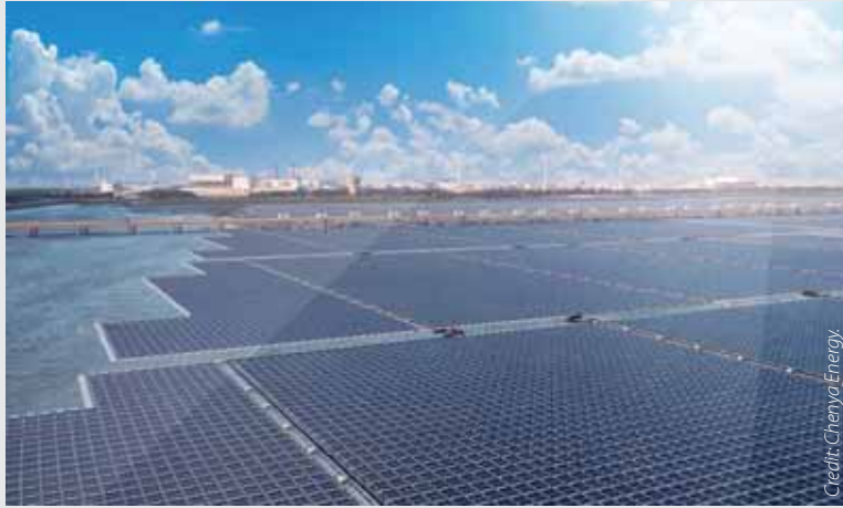
The 181MWp project from Chenya Energy Project was completed last November
